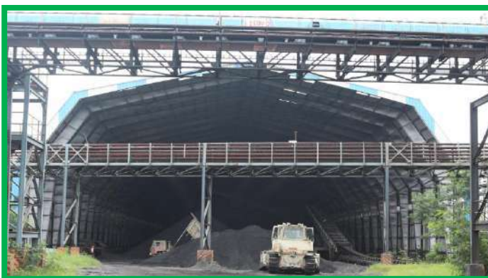
Coal Storage Shed: 10000 Tonne
