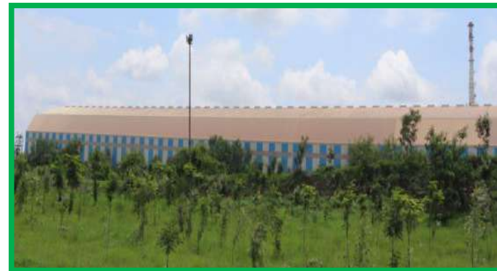
Limestone Storage Shed: 50000 Tonne
