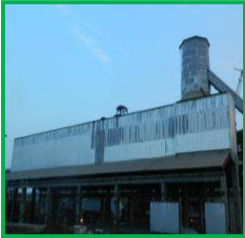
Gypsum Storage shed: 5000 Tonne
