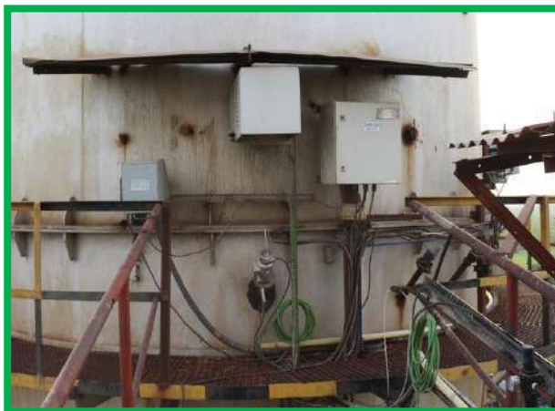
RABH CEMS and Opacity Meter installed at CPP stack and Server Room
