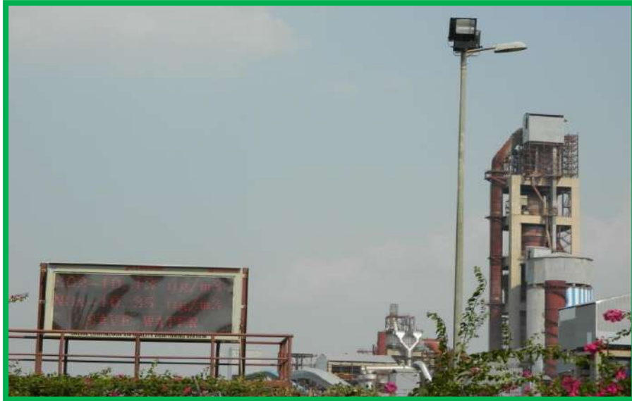
Data Display board at Plant Main gate
