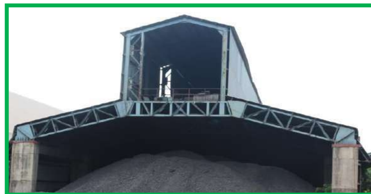
Additives Storage Shed: 15000 Tonne
