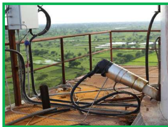
CPP CEMS and Opacity Meter installed at CPP stack and Server Room
