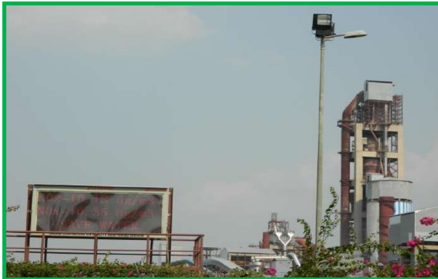
Data Display board at Plant Main gate
