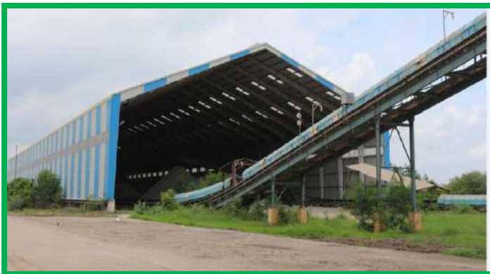
Slag Storage Shed: 10000 Tonne
