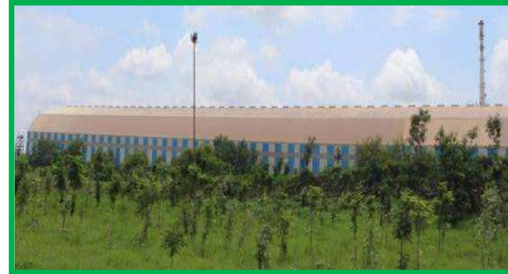
Limestone Storage Shed: 50000 Tonne
