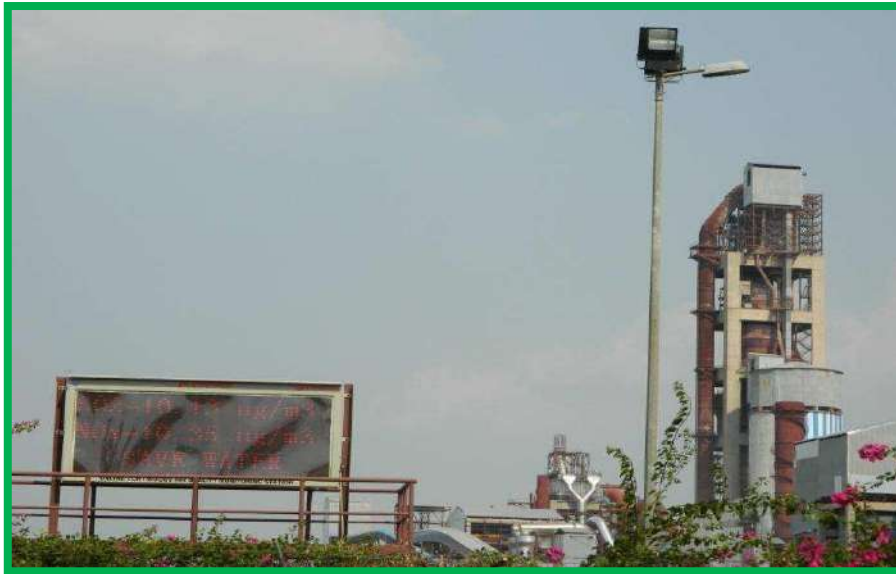
Data Display board at Plant Main gate
