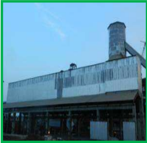
Gypsum Storage shed: 5000 Tonne
