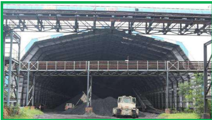
Coal Storage Shed: 10000 Tonne
