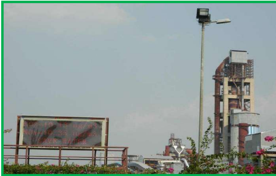
Data Display board at Plant Main gate
