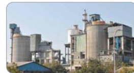
Kalol Grinding Unit Commissioned-0.5 Mn MT, Total Capacity-4.7 Mn MT
