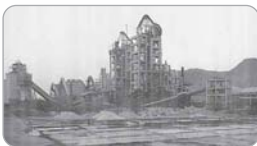
1st Integrated Plant at Sirohi, Total Capacity-0.5 Mn MT
