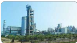
2nd Integrated Plant at Durg-1.8 Mn MT, Total Capacity-7.7 Mn MT
