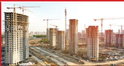
Concrete work for high rise towers and apartments
