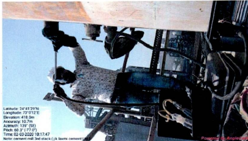
Cement Mill No.3 [24*41'29"N 73*0'12"E]
