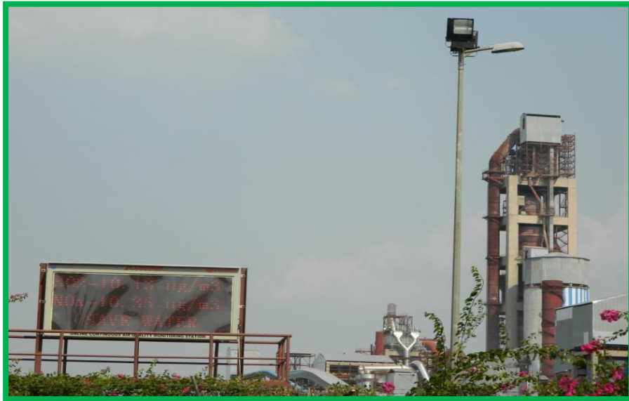
Data Display board at Plant Main gate
