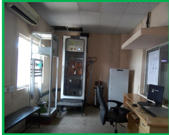
RABH CEMS and Opacity Meter installed at CPP stack and Server Room
