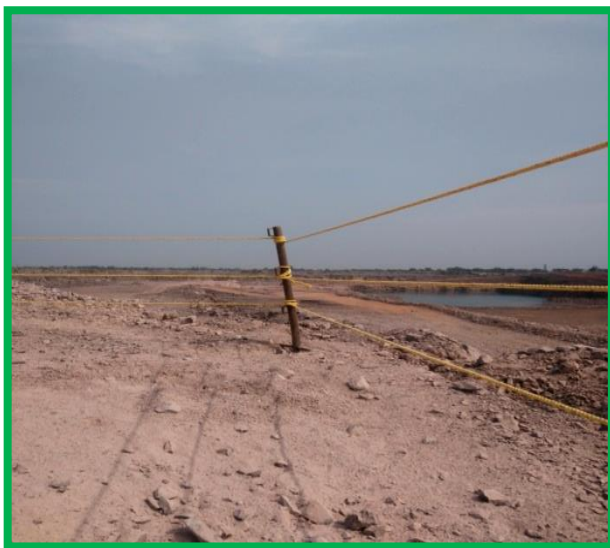
All bench edges are being fenced with rope and Steel pipes to check fall of men during Blast Hole Drilling and Blast Hole charging Operations.
