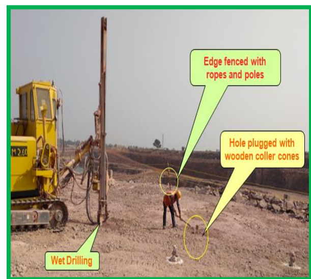
Wet drilling is being practiced regularly to control dust emission
