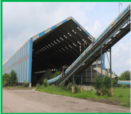
Slag Storage Shed: 10000 Tonne
