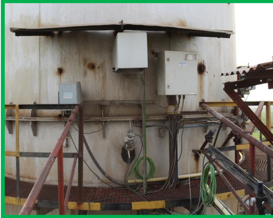
RABH CEMS and Opacity Meter installed at CPP stack and Server Room
