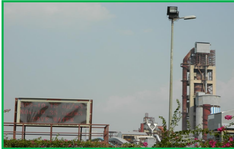
Data Display board at Plant Main gate
