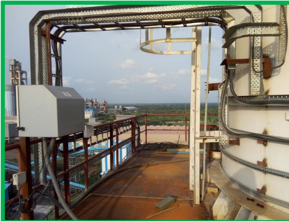
CPP CEMS and Opacity Meter installed at CPP stack and Server Room
