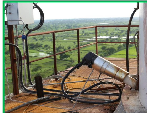
CPP CEMS and Opacity Meter installed at CPP stack and Server Room
