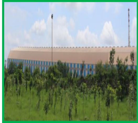
Limestone Storage Shed: 50000 Tonne
