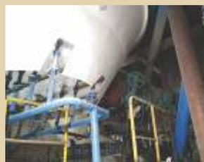
Solid Flow feeder installation in one of the Silos, to take Flyash in Cement Mill discharge, helps improve productivity and Flyash storage capacity.
