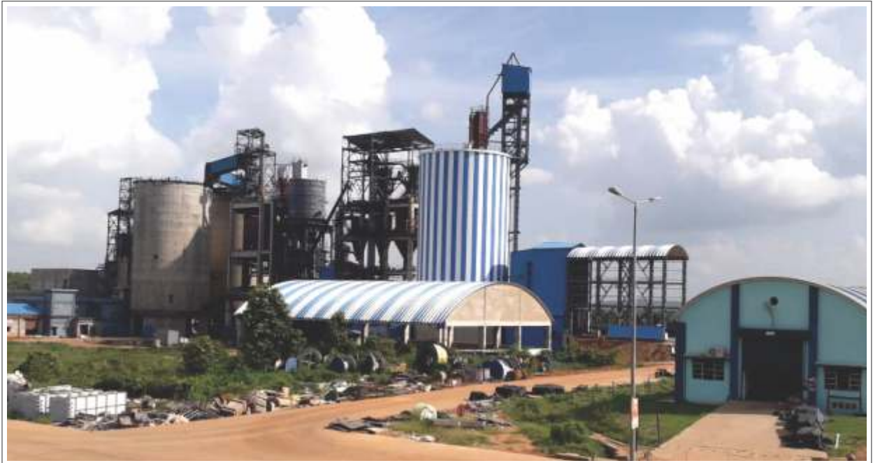
Cement Grinding Unit, Cuttack Odisha
