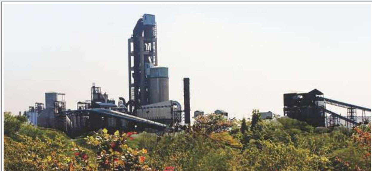
Integrated Cement Unit, Durg
