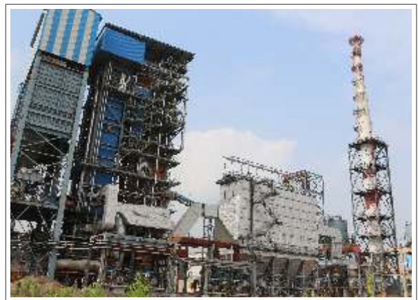
Thermal Power Plant - Durg
