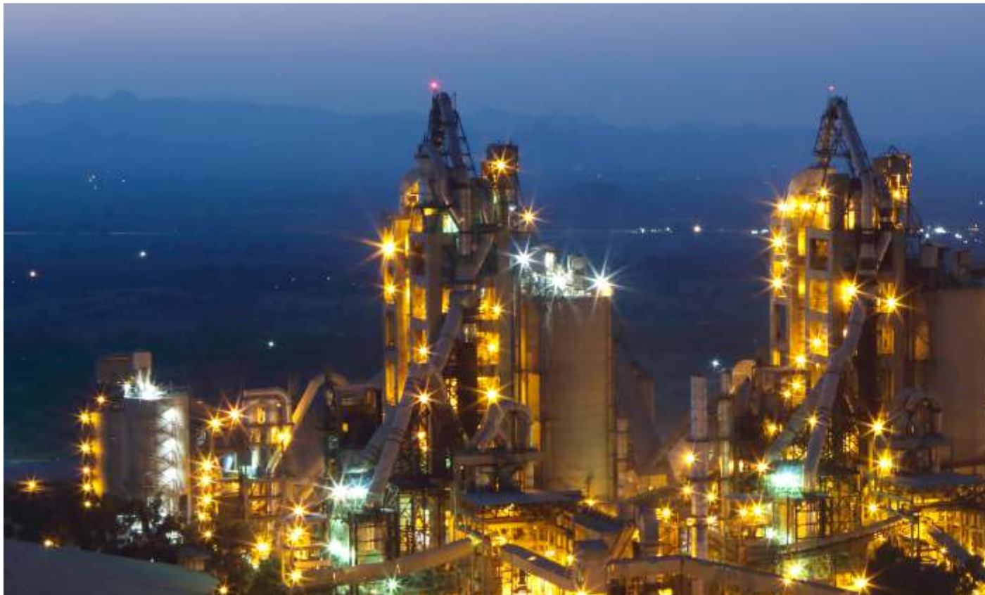
Integrated Cement Unit, Sirohi
