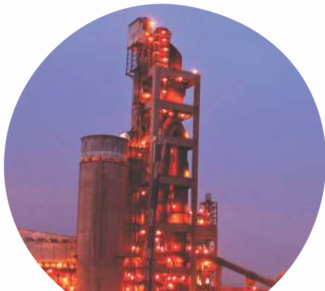
INTEGRATED CEMENT UNIT AT DURG
