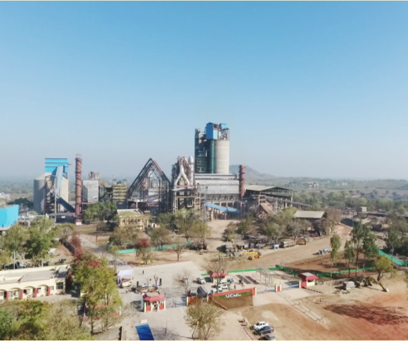
A view of UCWL's Integrated Cement Plant
