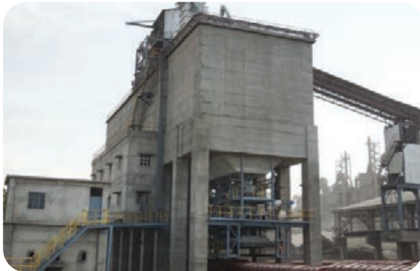
Automated wagon clinker loading unit, Sirohi
