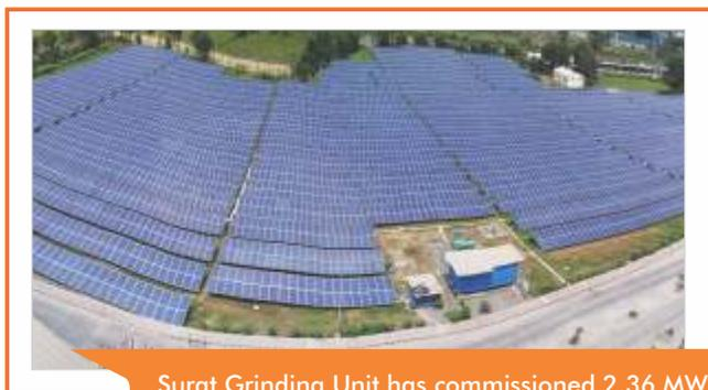
Surat Grinding Unit has commissioned 2.36 MW captive solar power plant that meets about 12 % of the total power requirement of the Unit
